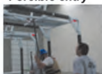
Ceiling breach and pull
