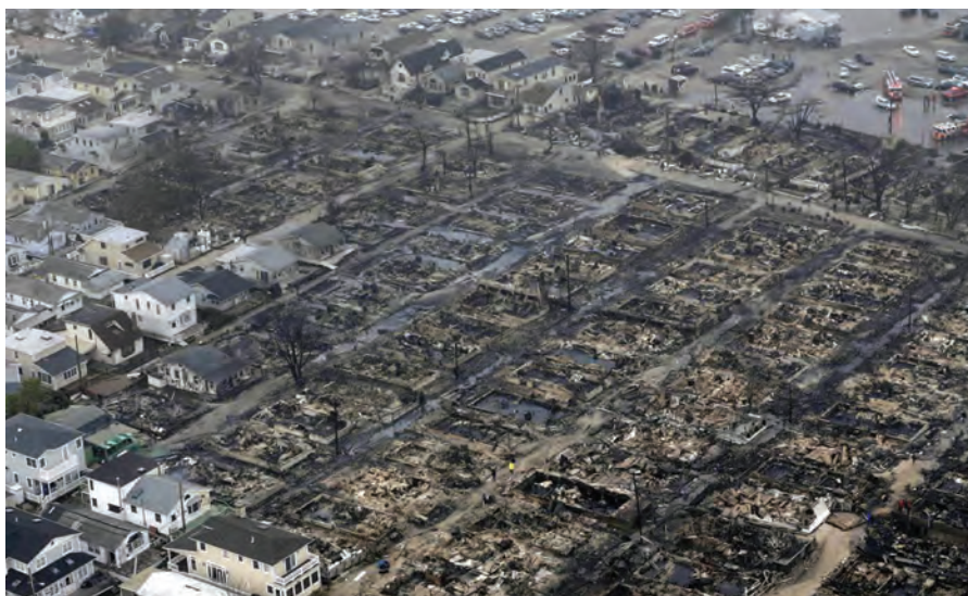
Flood and fire damage caused by Sandy
